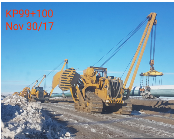
15. Excavator clearing ditch – Km 99+100 – Nov 30, 2017
