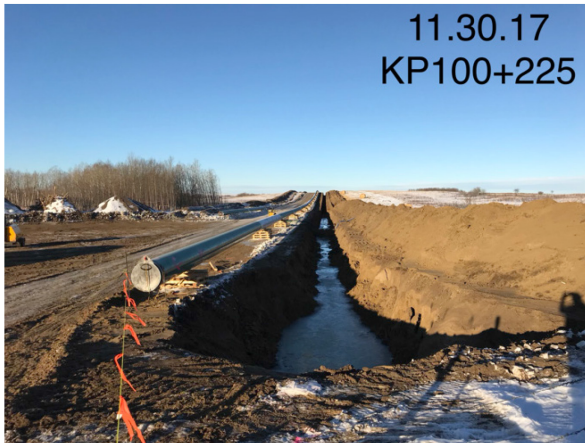
17. Ditch and pipe – km 100+225 – Nov 30, 2017
