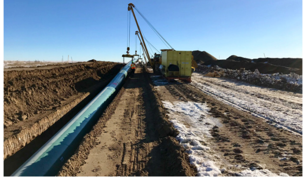
14. Lowering – in – km 99+050 – Nov 30, 2017
