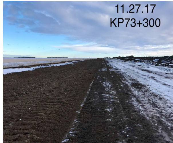
2. Backfilled Mainline – Km 73+300 – Nov 27, 2017
