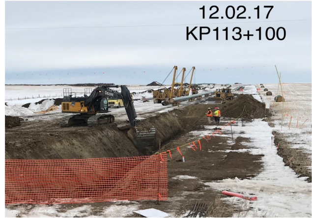
20. Bell hole work – Km113+100 – Dec 2, 2017
