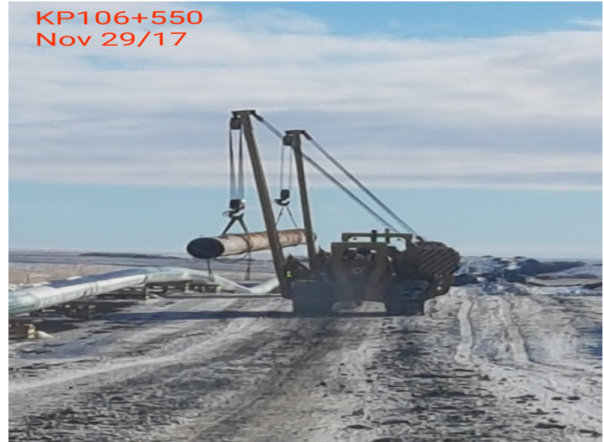
8. Side booms moving pipes – km 106+550 – Nov 29, 2017
