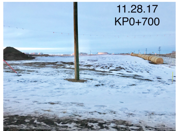
4. Completed work – Km 0+700 – Nov 28, 2017
