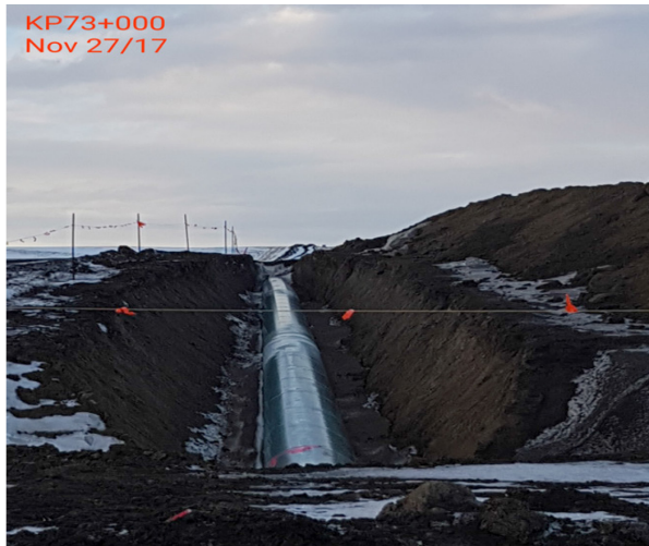
1. Tie-in work – Km73+000 – Nov 27, 2017
