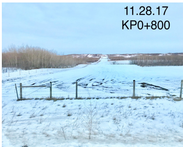
5. Completed Work – km0+800 – Nov 28, 2017
