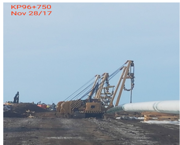
6. Pipe lowering in – Km 96+750 – Nov 28, 2017
