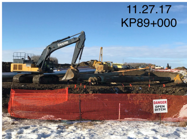
3. Tie-in work – Km 89+000 – Nov 27, 2017
